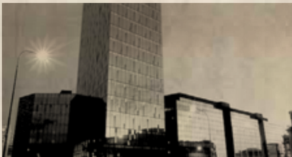
The Hamburger Factory Reykjavík Höfðatorg Tower. Groundfloor.
